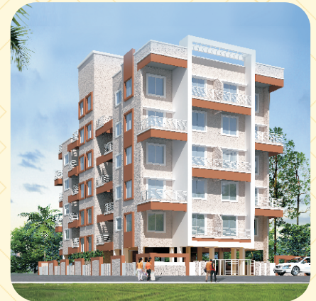
Shivansh Residency (Kiwale, Pune)
